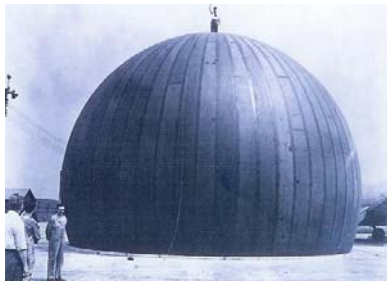
Figure 4 - The first radome prototype (1948). Walter Bird stands on top (Topham, 2002)
